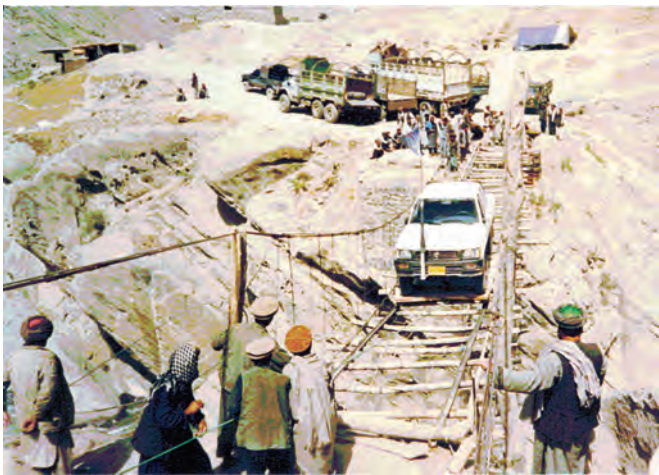
Passage between Fayzabad en Talogan in the North of Afghanistan. Trucks are unloaded at one side of the temporary bridge. Goods are placed on pallets and pulled to the other side. Maximum capacity is 1.000 kg but exceptions are made for 4WD vehicles, preferably without drivers behind the wheel!
